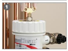
With a standard radiator key, remove the Pro-Fill air vent. The built-in, one-way, valve will prevent water from escaping. Attach chemical adaptor and feed in chemical.
