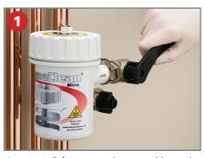
Important – Before commencing any servicing work, turn off electrical supply to the boiler. Ensure the water is not too hot to undertake work on the system. Turn off both isolation valves to the marked OFF position. Loosen the air vent to release internal pressure. When venting, protect the surface below the canister with a dust sheet or container to capture any drops of water.
