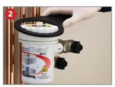
Using the MagnaClean Micro lid spanner, carefully unscrew the lid.
