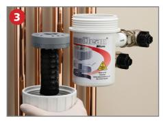
Remove the complete lid assembly from the MagnaClean Micro. Turn the lid assembly upside down in order that the underside of the lid acts as a drip tray.
